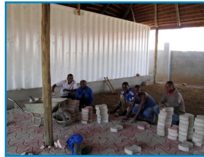
The Crew Laying Pavers
