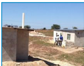
ACU Chisamba Campus Construction
