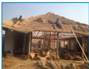
Olive Doke Pavilion Construction
