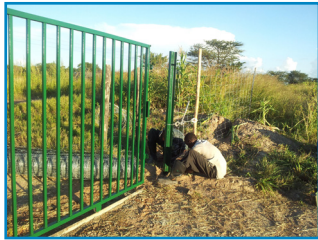
Gate installation at Chisamba
