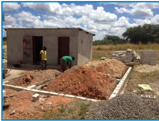
Caretaker's house under construction
