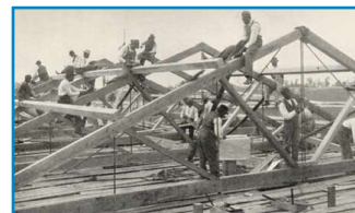
Tuskegee Institute - Student's helping in construction
