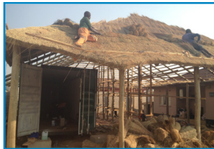
Construction of the ACU Olive Doko Pavilion
